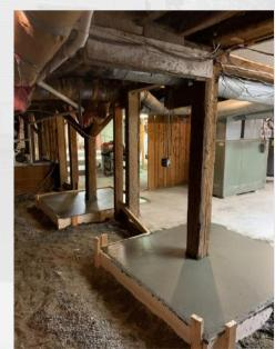
New concrete has been poured to support twenty support posts, strengthening The Pierce Block for years to come
